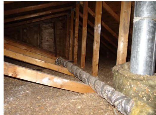
Photos 26 and 27: Bathroom exhaust vent and plumbing stack in attic space
