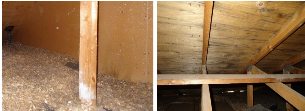
Photos 20 and 21: Moisture stains on gypsum board and framing members
