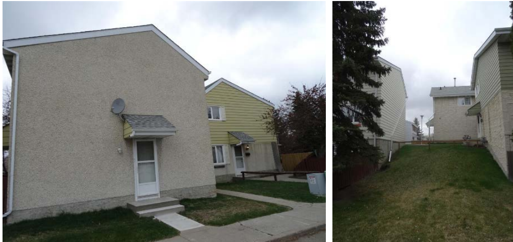
Photos 5 and 6: Stucco and metal siding installed to building block wall surfaces
