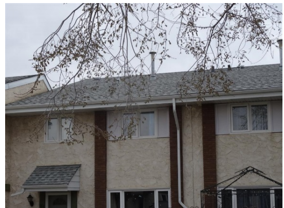
Photos 3 and 4: Wood trim boards and brick cladding at various wall surfaces
