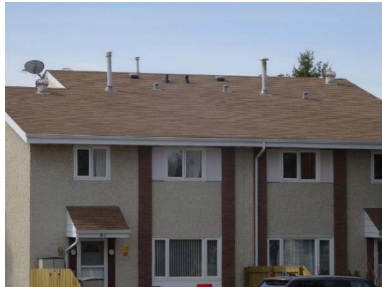
Photos 9 and 10: Asphalt shingles applied to upper and intermediate roof levels of complex
