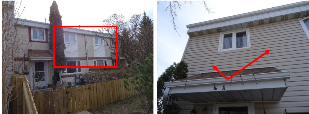
Photos 51 and 52: Vinyl siding at Units 2B, 2D, and Unit 4A where stucco replaced
