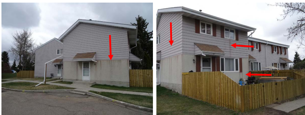
Photos 45 and 46: Stain marking of stucco finish surfaces at Building Block 7
