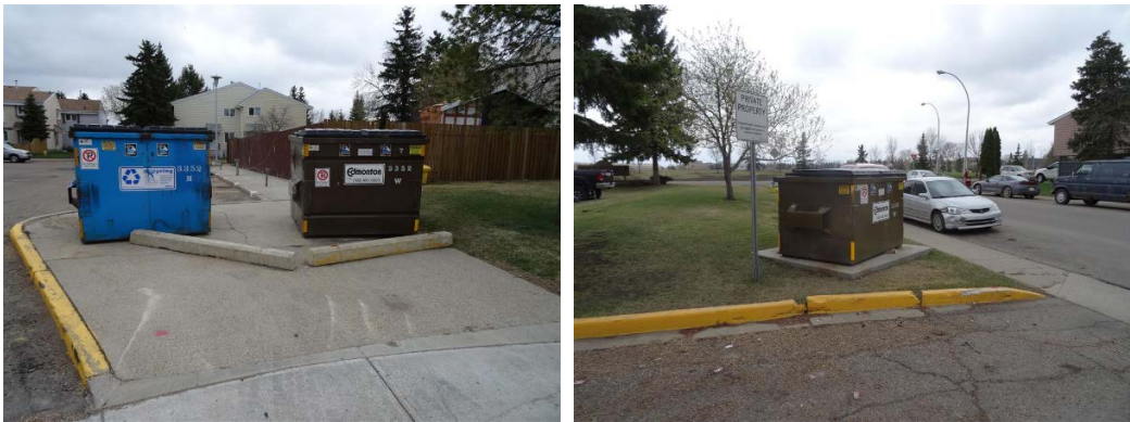
Photos 82 and 83: Concrete slabs for refuse bins on southwest and northwest side of site
