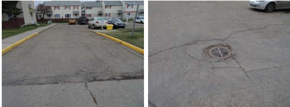
Photos 91 and 92: Pavement condition at south and southwest parking lot catch basin
