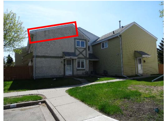
Photos 47 and 48: Stain marking of stucco at Building Blocks 6 and 21
