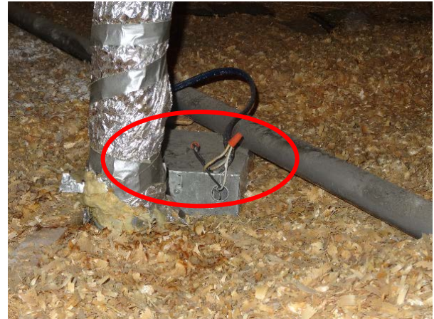
Photo 24: Corrosion at flue seam Photo 25: Unsecure electrical box and exposed wires
