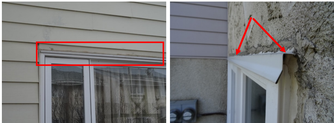
Photos 69 and 70: Caulking bead applied to head flashing joint above suite windows
