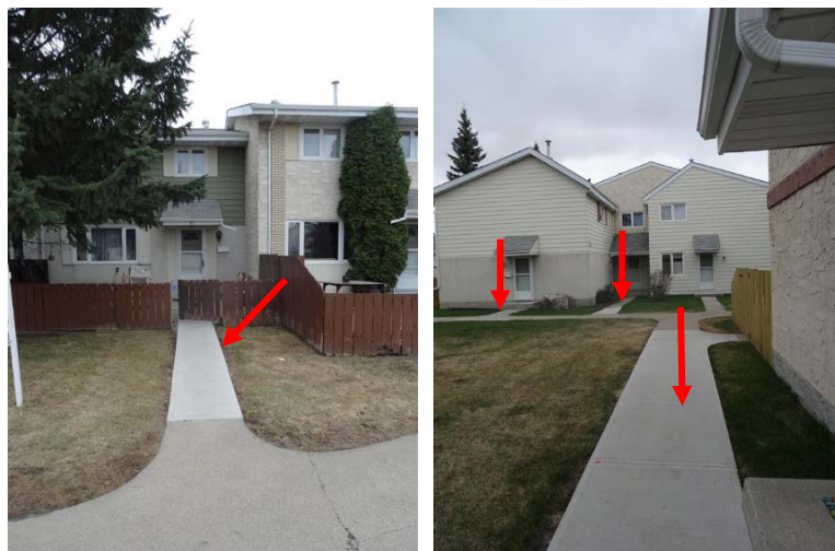
Photos 76 and 77: Newly installed concrete sidewalk pads at site
