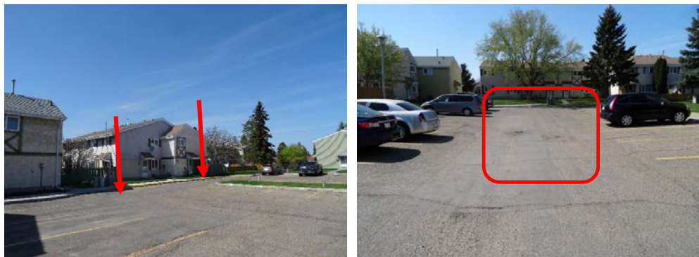
Photos 95 and 96: Patch repairs to pavement at southeast and northeast parking lots
