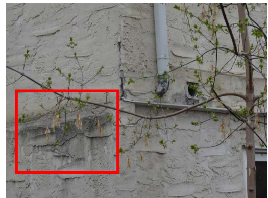
Photos 49 and 50: Stain marking below window and delamination near downspout at 9A
