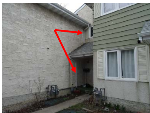
Photos 38 and 39: Downspout extensions routed internally at Building Block 9
