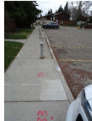
Photo 112: Newer concrete repair where pedestal located at northwest parking lot
