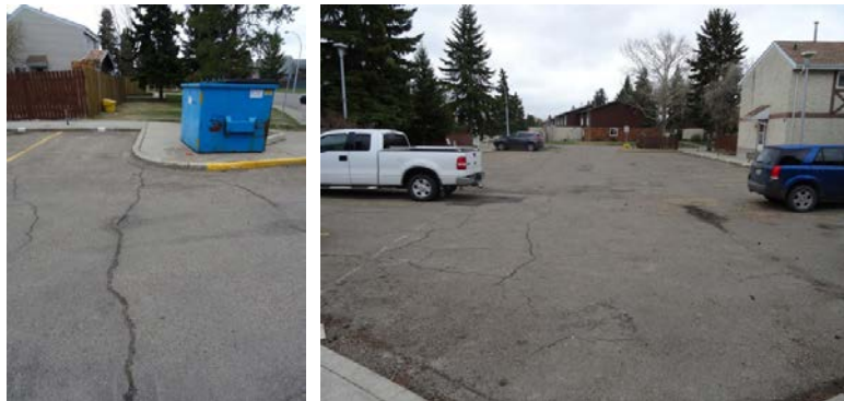
Photos 93 and 94: Transverse crack and deteriorated pavement at northwest parking lot
