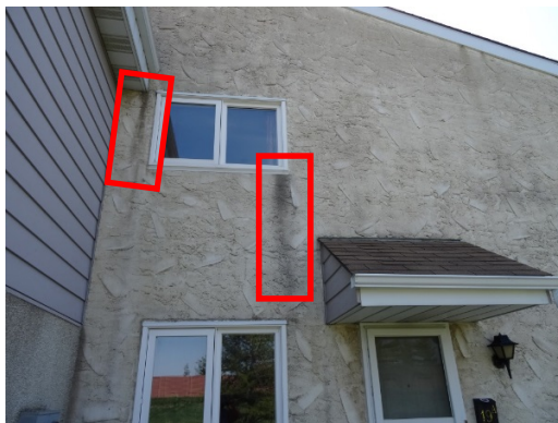
Photos 49 and 50: Stain marking below window and delamination near downspout at 9A
