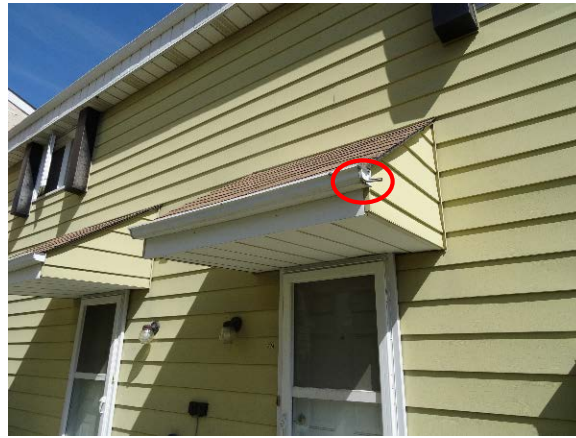
Photo 40: Grommet sleeve used to drain entry roof
