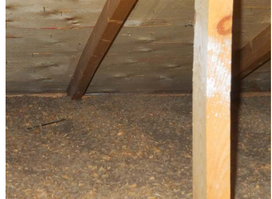
Photos 16 and 17: A combination of blown in insulation and wood shaving in attic spaces
