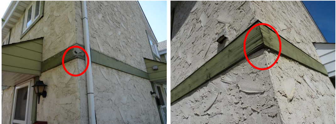
Photos 54 and 55: Deterioration of wood trim boards at various wall regions
