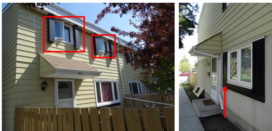
Photos 59 and 60: Metal rim at 2 nd floor regions and shutters at main floor window
