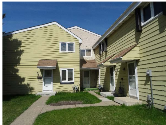
Photos 11 and 12: Asphalt shingles applied to shed style roofs above unit entries
