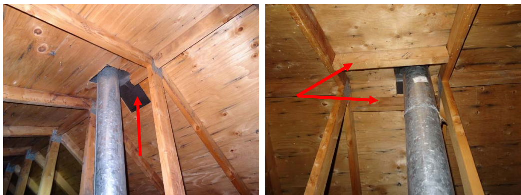
Photos 22 and 23: Roof framing cut or modified at Units 4A and 5D
