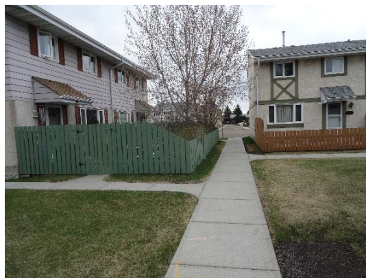
Photo 101: Green and cedar coloured stain finish applied to newer wood fencing
