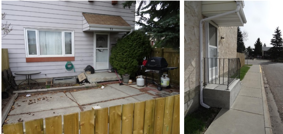
Photos 84 and 85: Concrete stoop and 3-riser steps at unit entries
