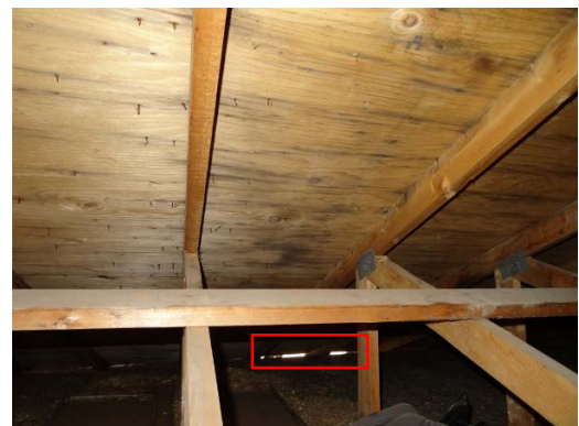
Photos 28 and 29: Moisture stained roof deck and daylight viewed at roof edge
