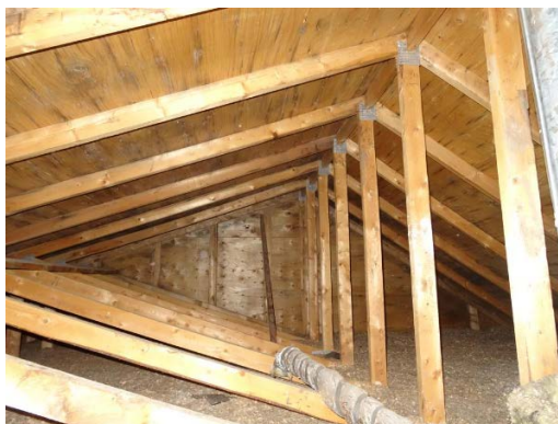
Photos 28 and 29: Moisture stained roof deck and daylight viewed at roof edge
