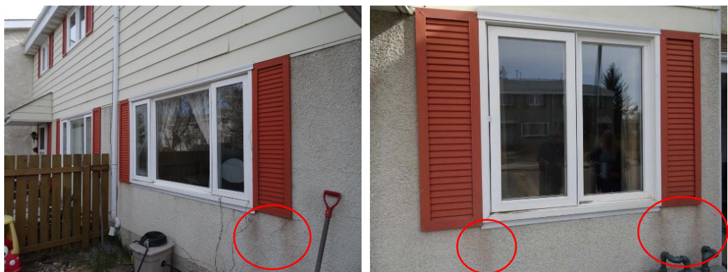
Photos 63 and 64: Stains at operable casement units on west and south sides of Unit 21C
