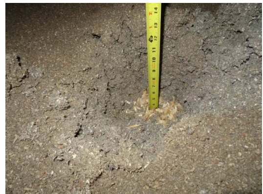
Photos 18 and 19: Blown-in cellulose over wood shavings within attic space
