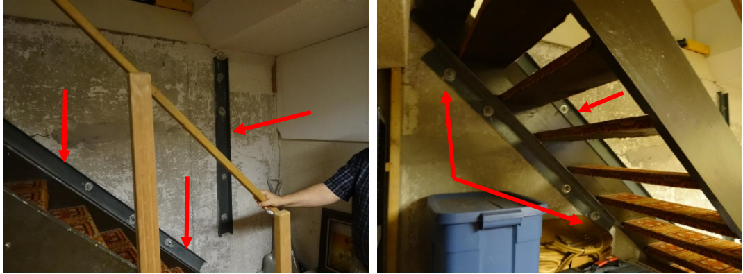
Photos 74 and 75: Steel framing members secured to basement foundation wall
