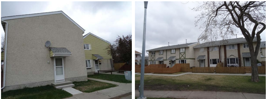
Photos 41 and 42: Stucco, metal siding, and brick veneer wall claddings at complex
