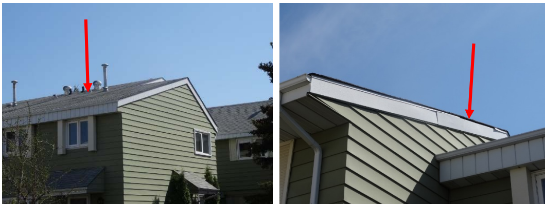
Photos 30 and 31: Curling of shingles and missing rake edge flashing above Unit 1F
