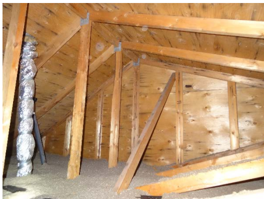
Photos 18 and 19: Blown-in cellulose over wood shavings within attic space
