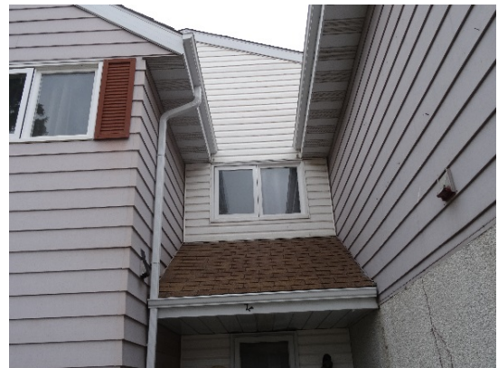
Photos 11 and 12: Asphalt shingles applied to shed style roofs above unit entries
