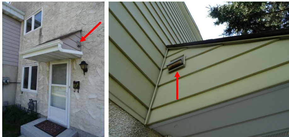
Photos 106 and 107: Blocked exhaust vents at unit entry canopies
