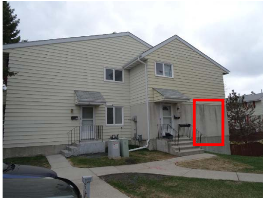
Photos 47 and 48: Stain marking of stucco at Building Blocks 6 and 21
