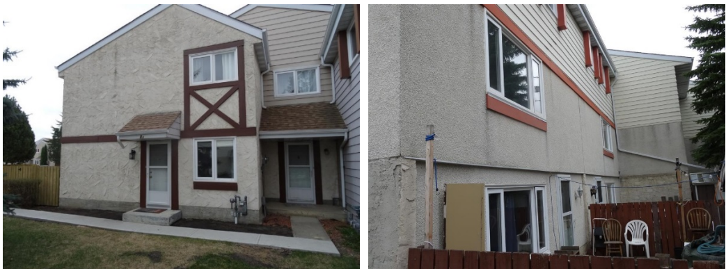
Photos 43 and 44: Wood trim boards and metal cladding applied to exterior walls
