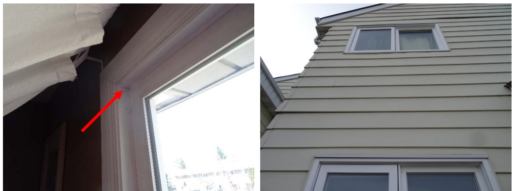
Photos 67 and 68: Stain at 2 nd floor window (Unit 4A) and loose siding (Unit 14C)
