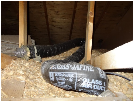
Photos 26 and 27: Bathroom exhaust vent and plumbing stack in attic space
