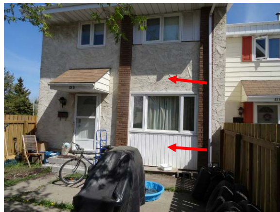
Photo 53: Original stucco and newer vinyl siding above at Unit 21D
