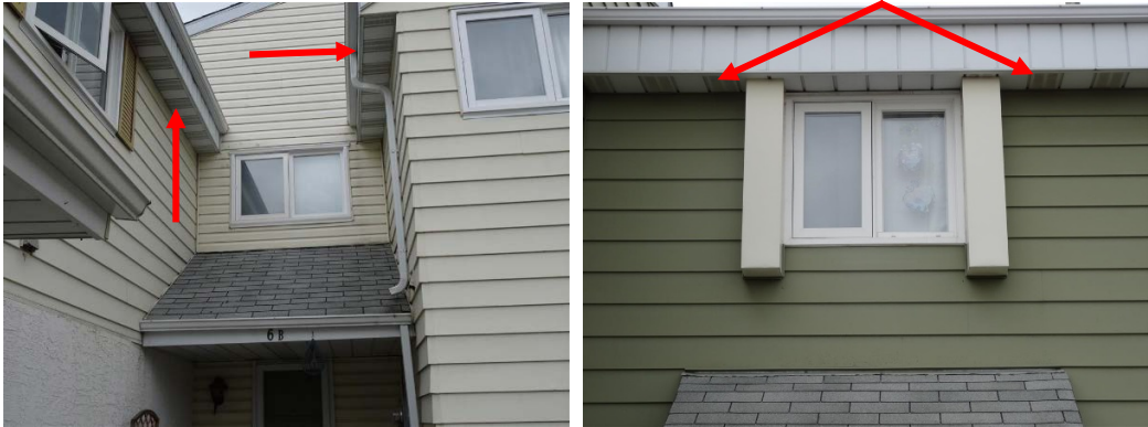
Photos 32 and 33: Soffit panels and vinyl siding used as a fascia trim at upper roof level
