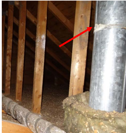
Photo 24: Corrosion at flue seam Photo 25: Unsecure electrical box and exposed wires
