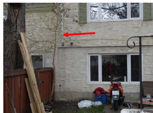
Photos 38 and 39: Downspout extensions routed internally at Building Block 9
