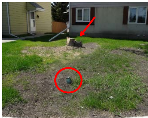
Photo 78: Tree stump and exposed shut-off valve
