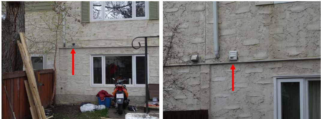
Photos 104 and 105: Missing cover and buildup of lint at dryer exhaust vents at Block 6
