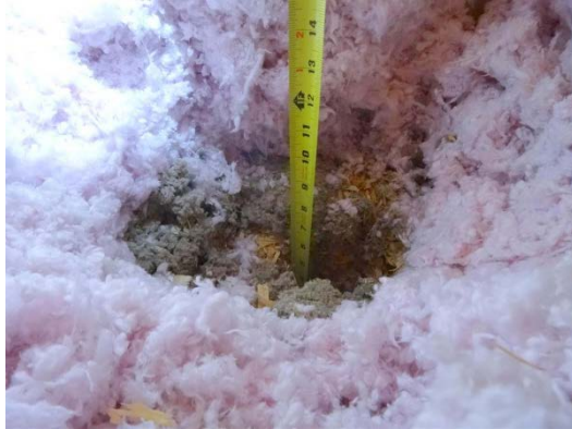
Photos 16 and 17: A combination of blown in insulation and wood shaving in attic spaces
