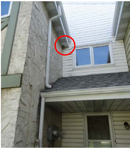
Photo 34: Stain marked soffit panels at intermediate roof level
